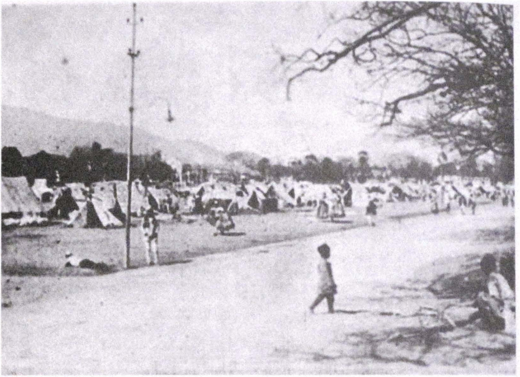
13. Shelters after the earthquake at Tundikhel
