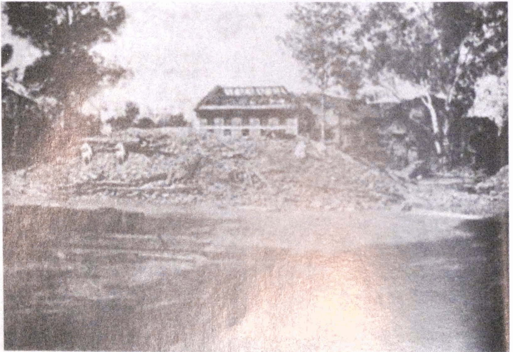
18. The Machhendranath Temple, Patan
