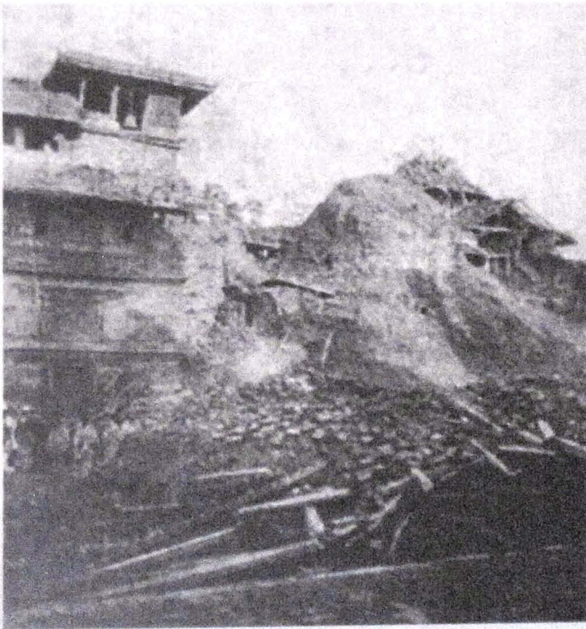
40. Degutale Temple after the earthquake
