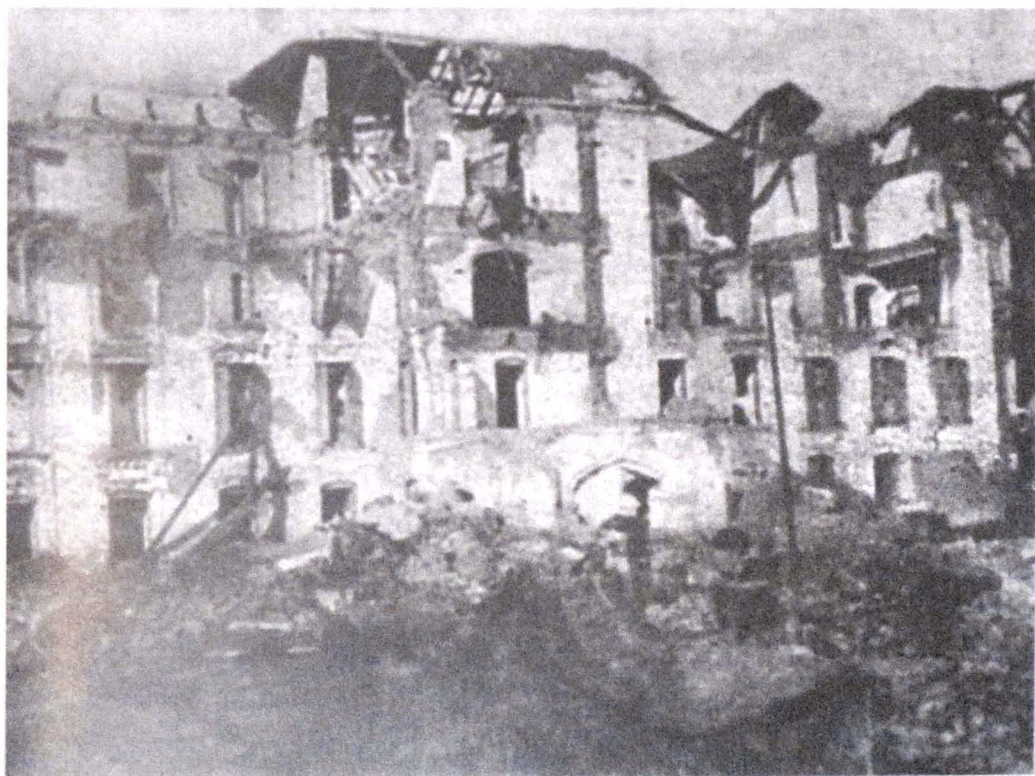
32. The Shital Niwas after the earthquake
