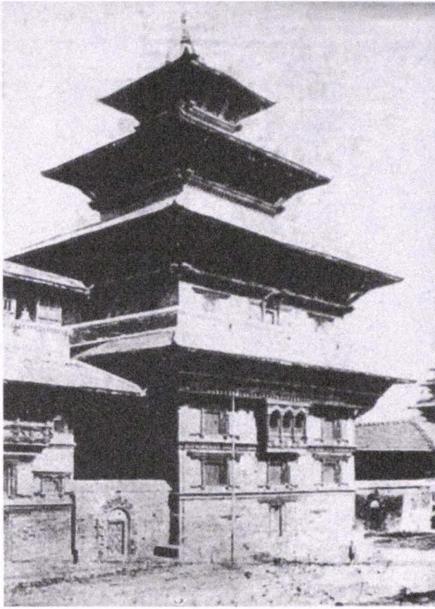
39. Degutale Temple, Patan, before the earthquake
