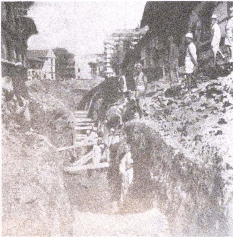
47. Sewage pipes being laid at New Road
