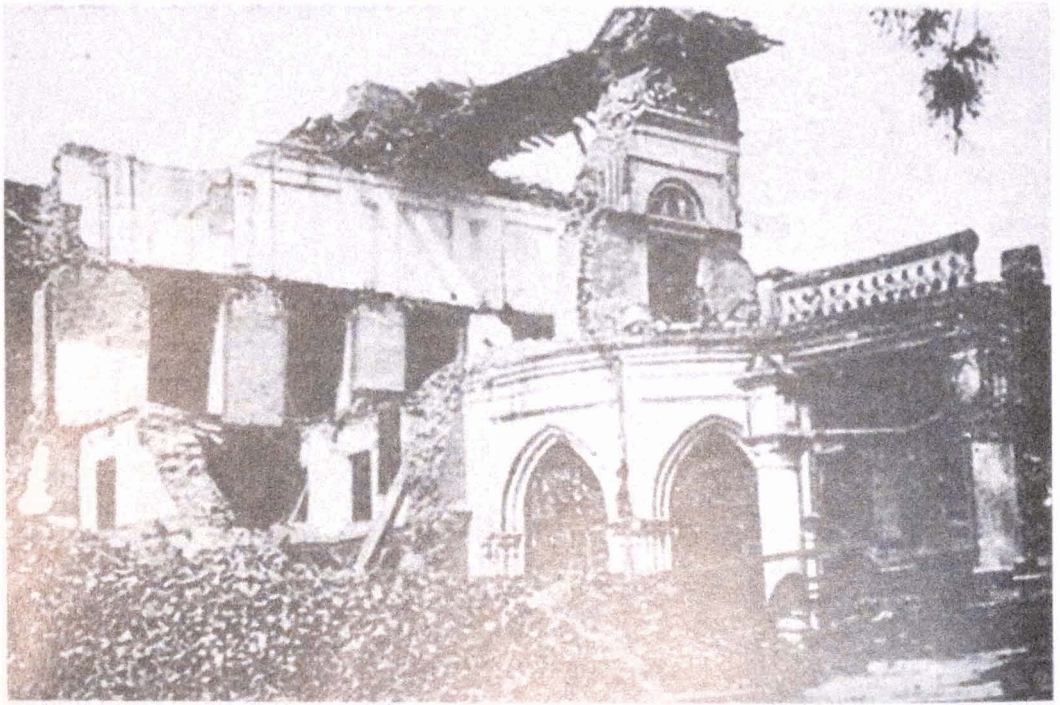
26. Gol Baithak after the earthquake
