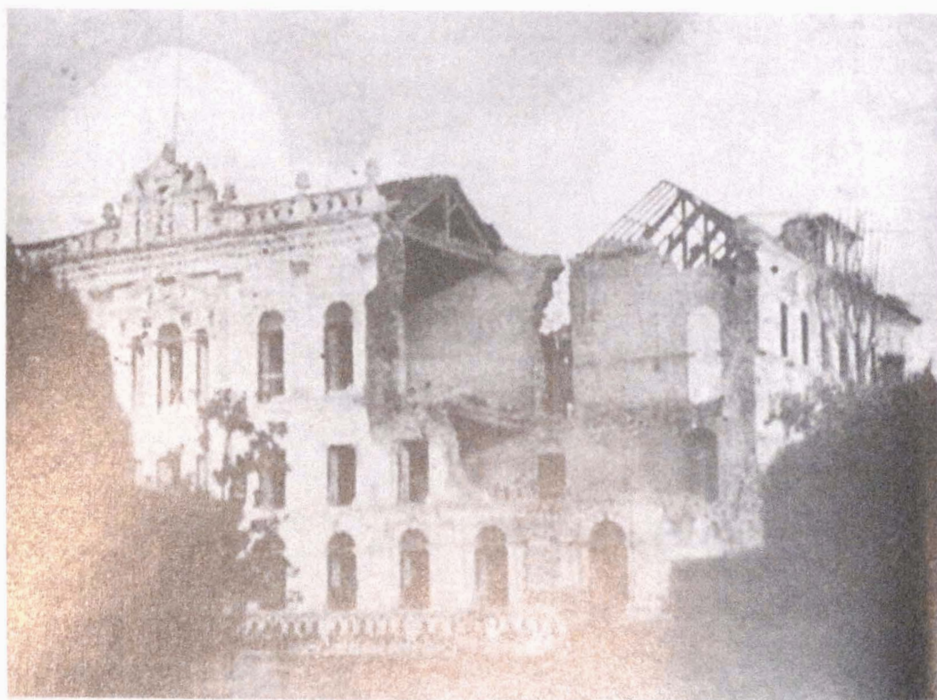
30. H.H. the Maharaja's palace after the earthquake
