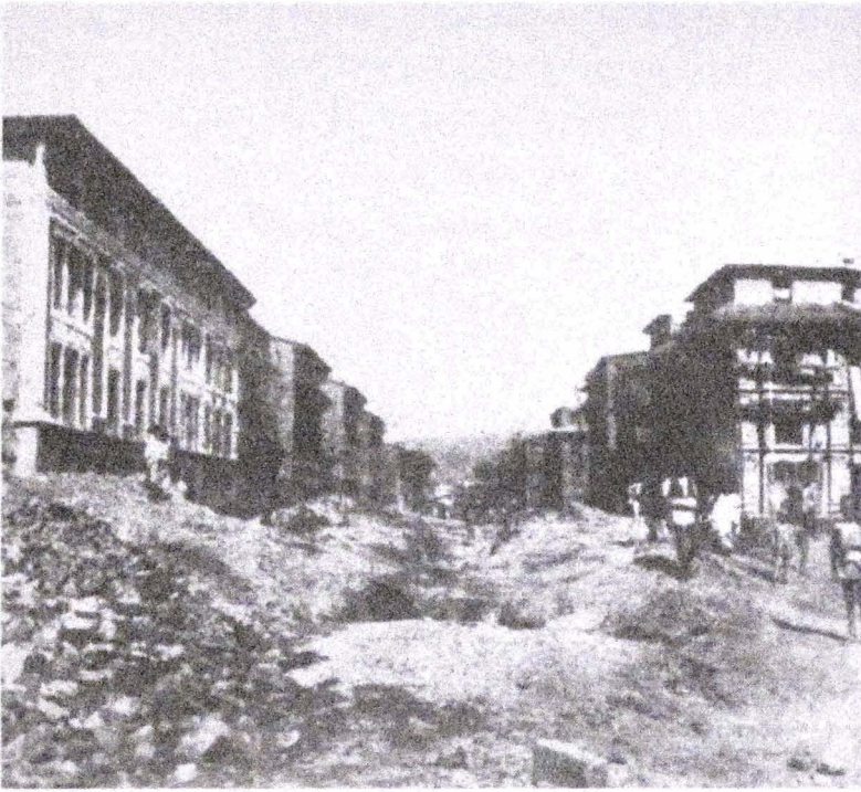
46. New Road from Hanuman Dhoka palace to Tundikhel under construction
